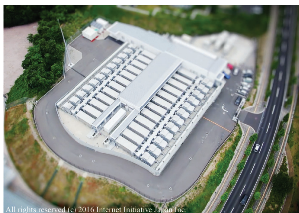
IMAGE 2.2 Example of a Data Center
